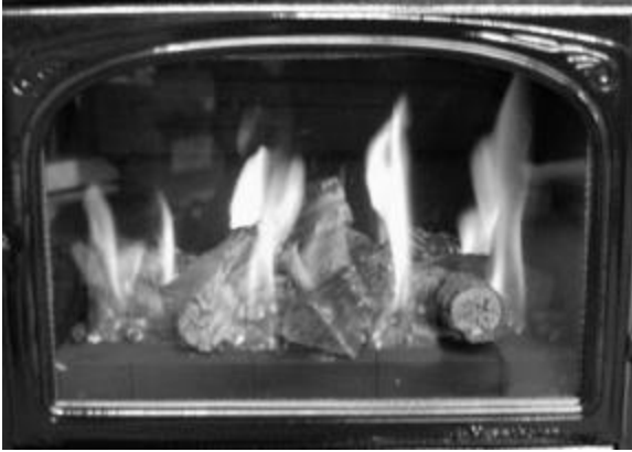
Figure 14 Typical Flame Pattern
